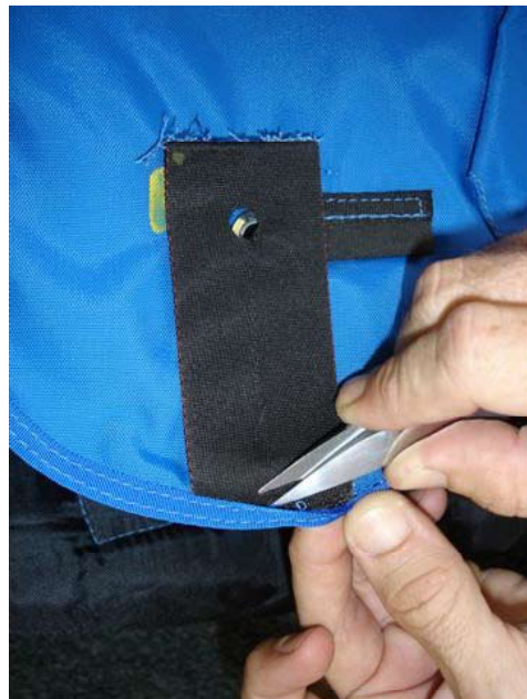
1.3 Carefully un-pick edge binding and cut TYPE 12 Webbing
